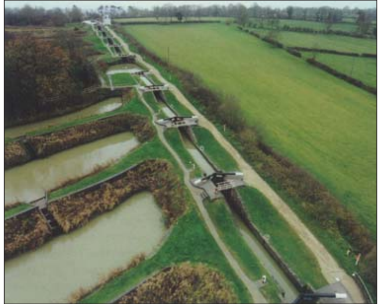
The Foxton flight of locks in rural Leicestershire. This important structure is designated as a conservation area and a management agreement has recently been developed for the site.
