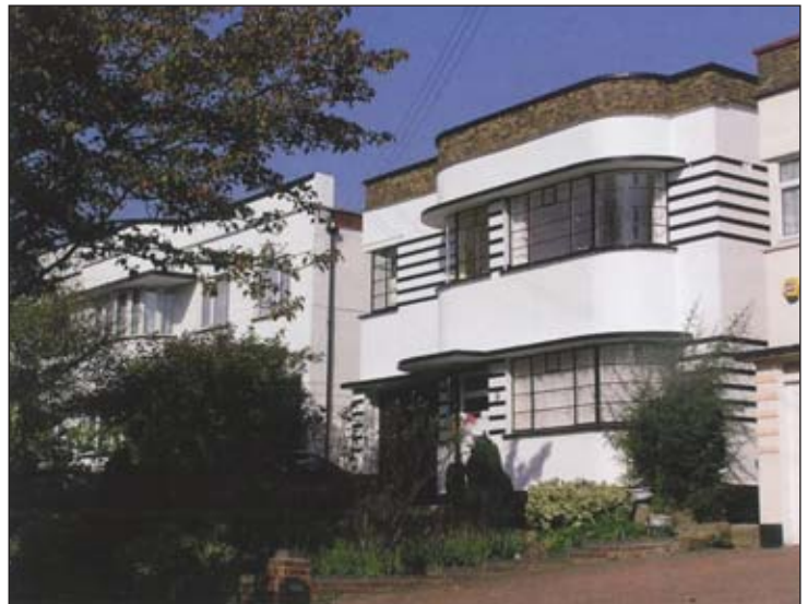
Abbotshall Avenue, Enfield - example of a locally listed modern building that adds significant value to its neighbourhood.
